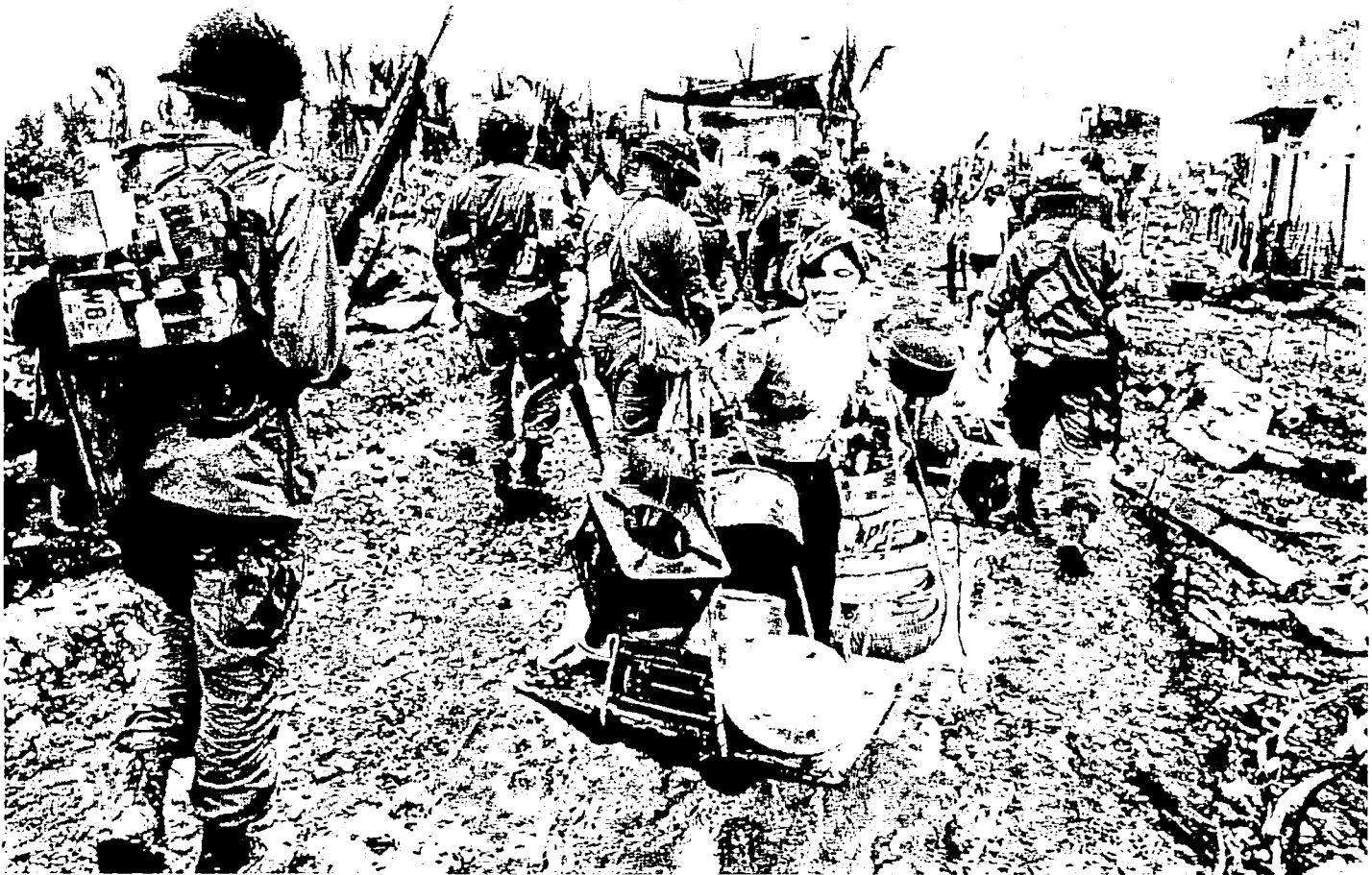
CARNAGE. Above, a scene from a Saigon neighborhood reduced to rubble after U.S. forces fought Viet Cong snipers there in 1968. Below, the aftermath of a car bomb in Baghdad's Karada neighborhood
